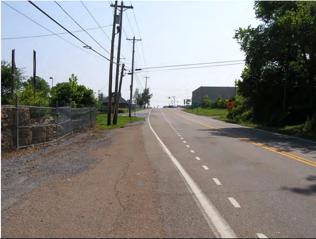
Photo 3: STA 404+00 LT (SR-1). View of SR-1 facing northeast.
