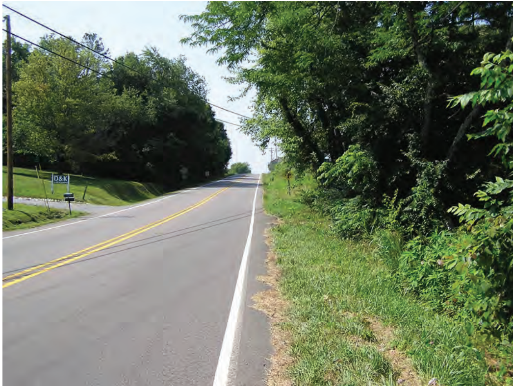
Photo 6: View from existing SR-2 ROW facing south towards proposed ROW.
